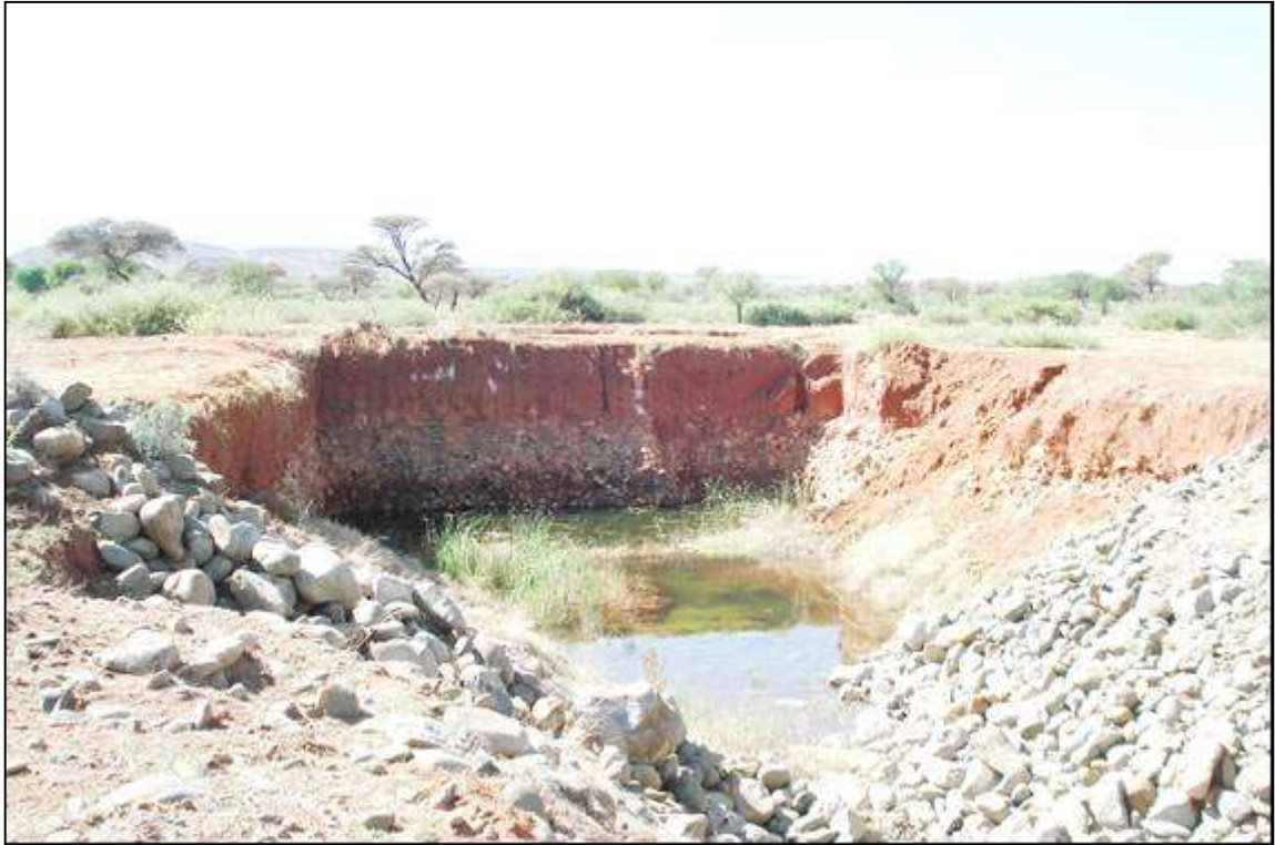
Photo 4. Non-rehabilitated pit by J. Crause. Overburden ~ 2 m, Gravel thickness ~ 2 m.
