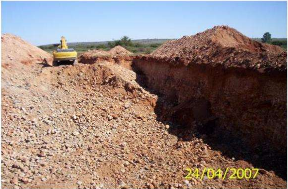
Photo 17. Pangea's bulk sampling site (Middelrand 820 HN) on Dry Harts terrace. Calcreted silt overburden ~ 1.5 m, poorly calcreted gravel ~ 2 m. Pangea reported second layer of gravels ~ 2 m thick near bedrock.
