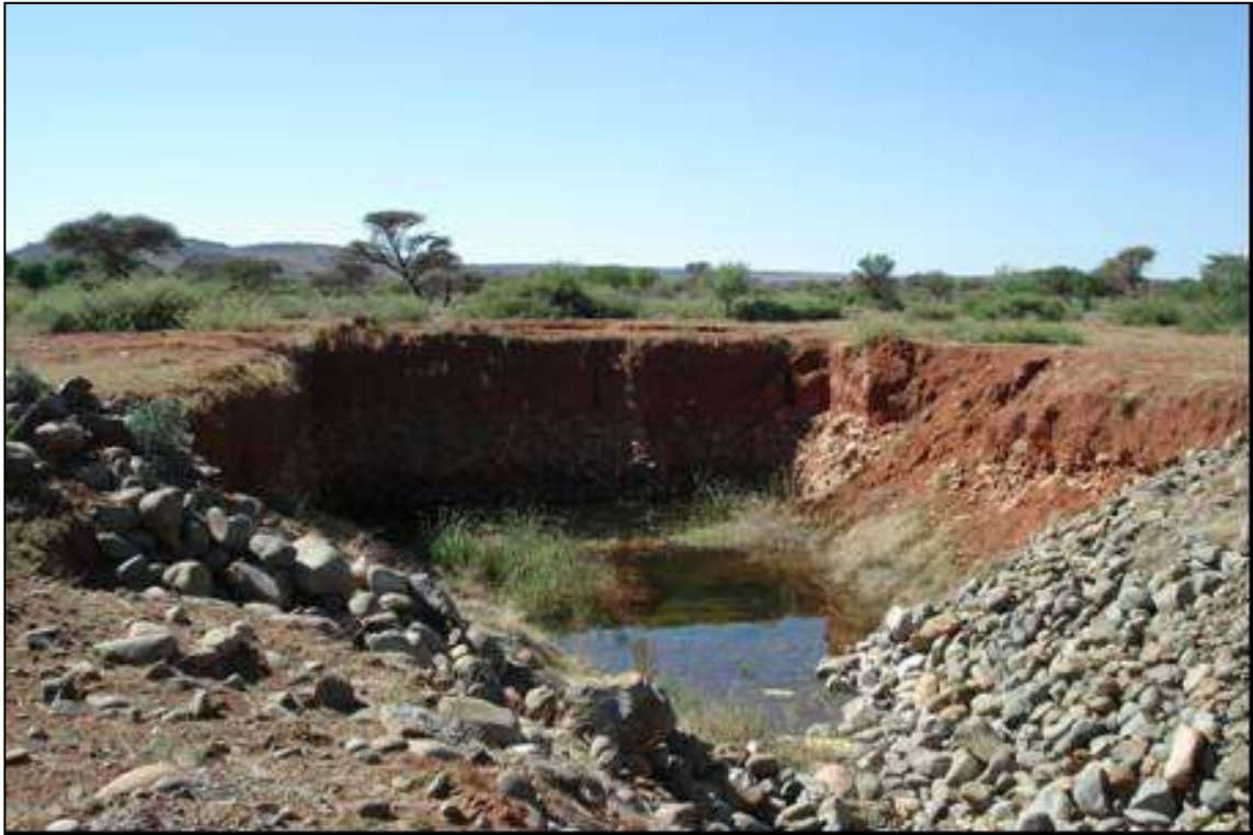
Photo 7. Not backfilled quarry left by Mr. J. Du Plooy. Overburden (soil, silty sand) ~ 2 m, gravel ~ 2.5 m.
